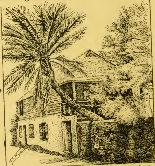
Before it was renovated
